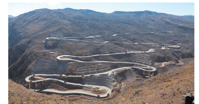
Road disaster prevention measures using the artificial slope stabilization method
