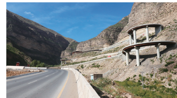
Curved steel box girder bridges built on steep slopes
