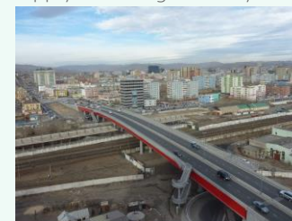
Mongolia – Narnii Zam (“Sun Road”), built within the scope of the Project for Railway Flyover Construction in Ulaanbaatar City
