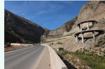
Pakistan – N-70 East-West Road Improvement Project
