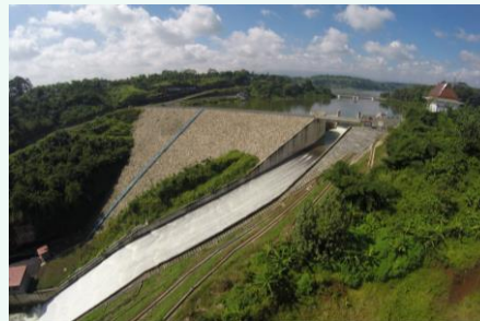
Indonesia – Jatibarang Dam, completed within the Integrated Water Resources and Flood Management Project for Semarang City
