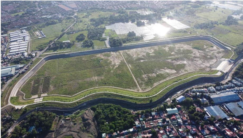
Imus Detention Basin (The Philippines' first detention basin facility, 6 months after construction)
