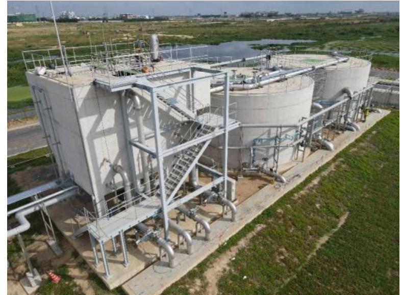
Exterior of the PTF treatment facility (Nov. 30, 2023)
