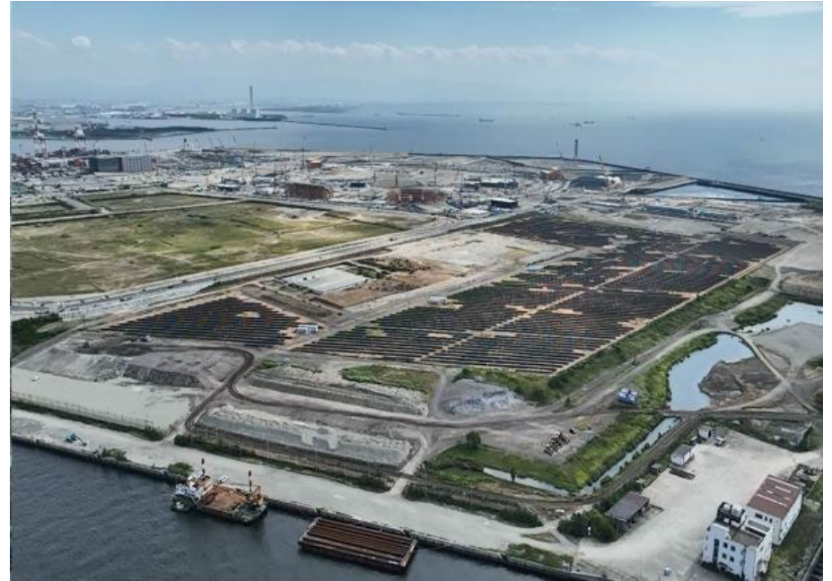
CM of parking lot construction work at the Japan Expo
