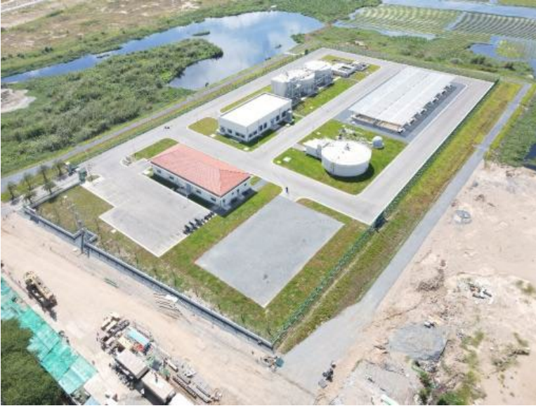
Completed sewage treatment plant (Nov. 30, 2023)
