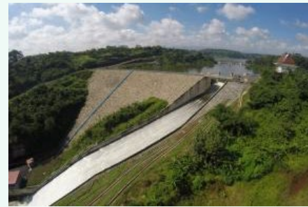
Indonesia – Jatibarang Dam, completed within the Integrated Water Resources and Flood Management Project for Semarang City
