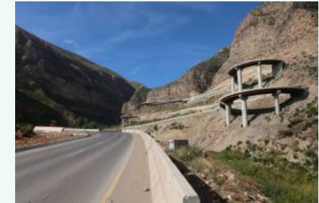
Pakistan – N-70 East-West Road Improvement Project
