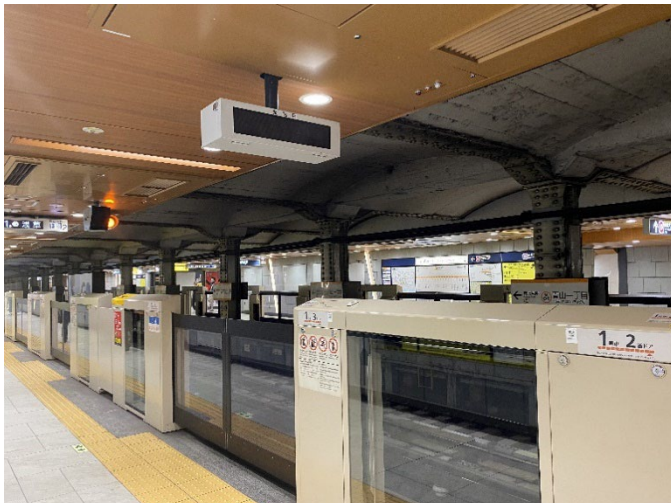
Fig. 9 Aoyama Ichōme Station on Ginza Line, 2020 – contrast between ceiling above the tracks and the platform
