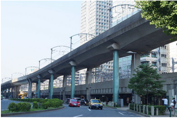
Fig. 10 Viaduct for Chūō Line at Tokyo Station (2000)
