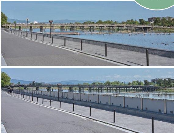
Top: Normal conditions (watertight barrier stored) Bottom: Flood conditions (watertight barrier deployed)
