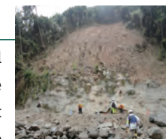
▲ An on-site field survey of collapsed land
