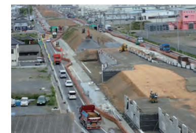
▲ A road project utilizing CM
