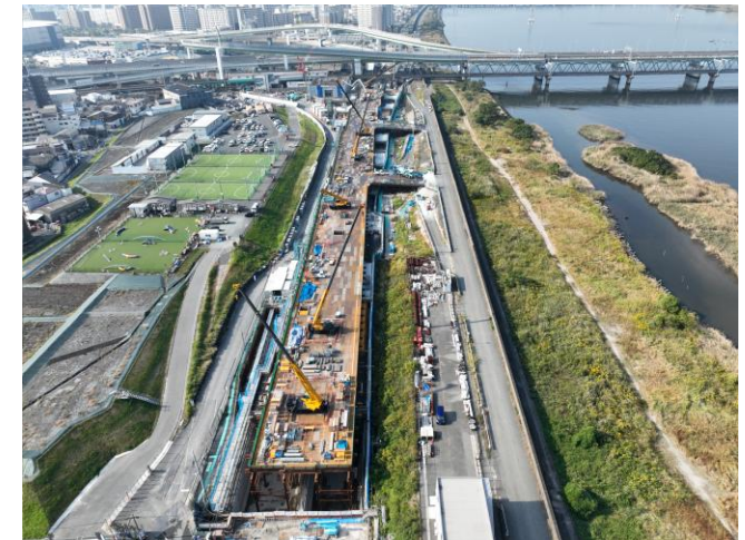
CM associated with embankment integrated road construction
