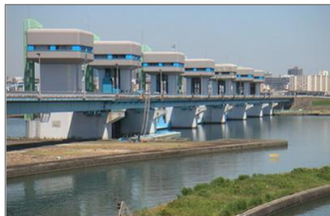
Yodo River, Yodo River system (Osaka City, Osaka Prefecture) (1971~1980)
