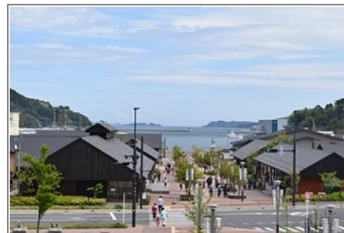
Onagawa Central District, Onagawa Earthquake Reconstruction Project (2013~2016)
