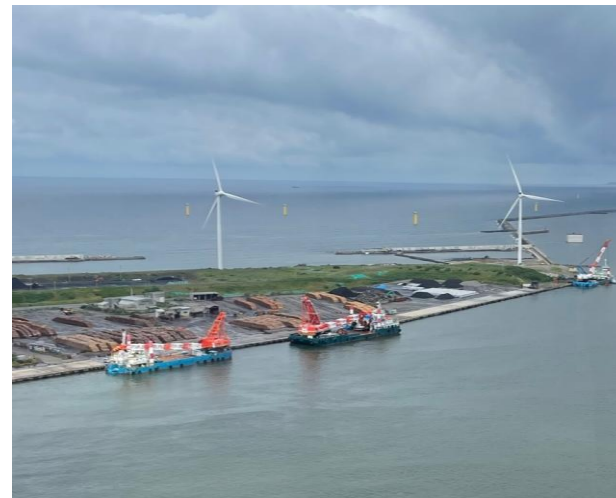
Offshore wind power generation business
