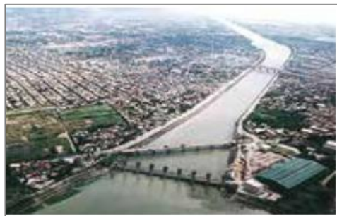
The Comprehensive Flood Control Project in Metro Manila (Philippines) (1977) Our first independent overseas business
