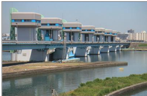
Yodo River, Yodo River system (Osaka City, Osaka Prefecture) (1971-1980)
