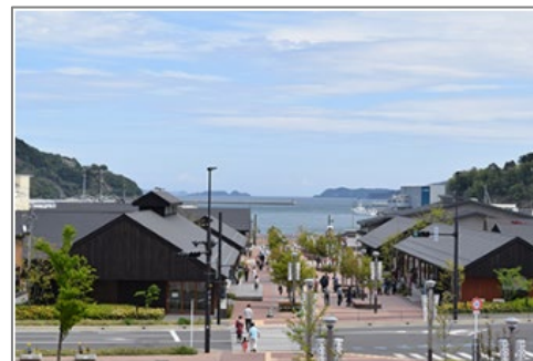
Onagawa Central District, Onagawa Earthquake Reconstruction Project (2013~2016)
