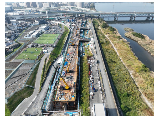
CM associated with embankment integrated road construction
