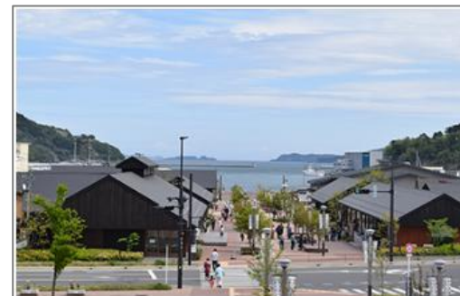
Onagawa Central District, Onagawa Earthquake Reconstruction Project (2013-2016)
