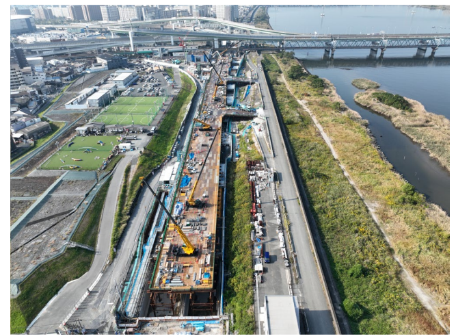
CM associated with embankment integrated road construction
