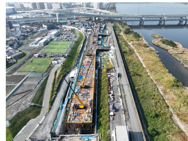
CM associated with embankment integrated road construction
